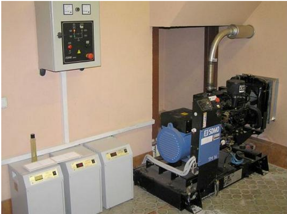
Fig. 8. Installation of compact diesel generator inside the substation building
